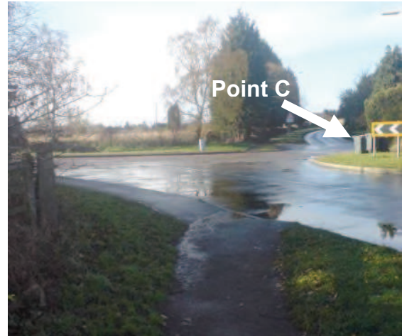
Looking west along Clophill Road towards the road junction and point C (behind bins and chevrons).
